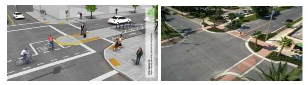
Figure 2: Median islands and curb extensions are two examples of traffic calming measures.
